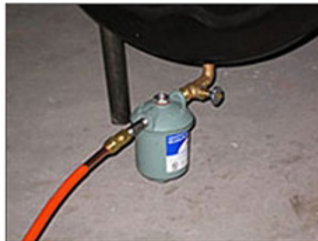
A proper new line and filter
